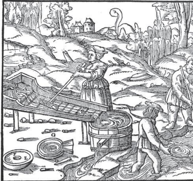
A—HEAD OF THE SLUICE. B—RIFFLES. C—WOODEN SCRUBBER. D—POINTED STICK.
